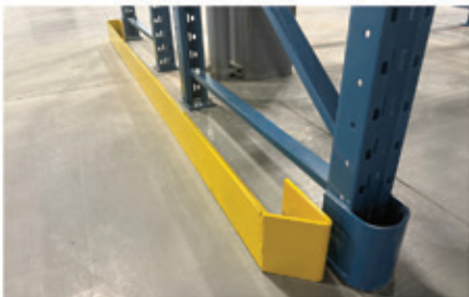
End of Aisle Guarding
